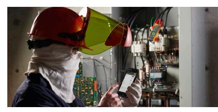
Fluke Connect allows measurements to be sent to a smartphone for logging, collaboration and analysis.
